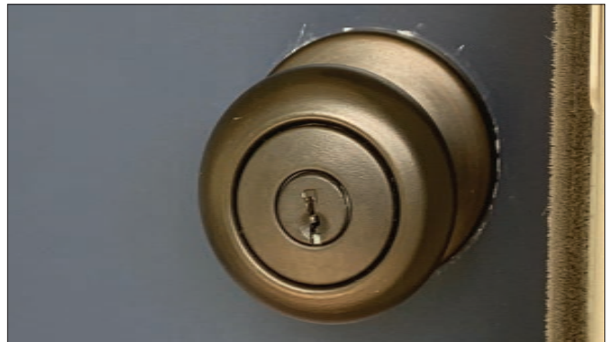
Finish damage caused by use
