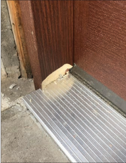
Defect to frame component due to improper handling
