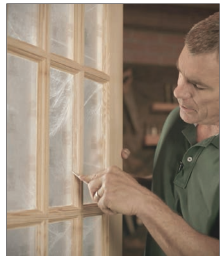
Removing glazing compound
