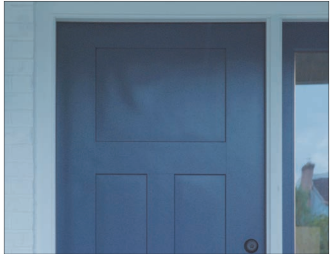
Bubble Defect (Fiberglass Door)
