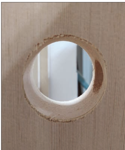
Blowout that can be covered by escutcheon
