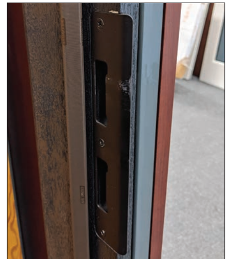
Acceptable hardware wear and tear
