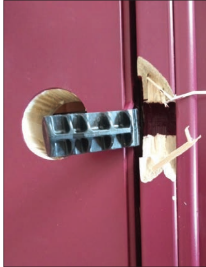
Defect to frame component due to improper handling
