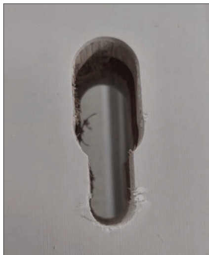
Blowout that can be covered by escutcheon
