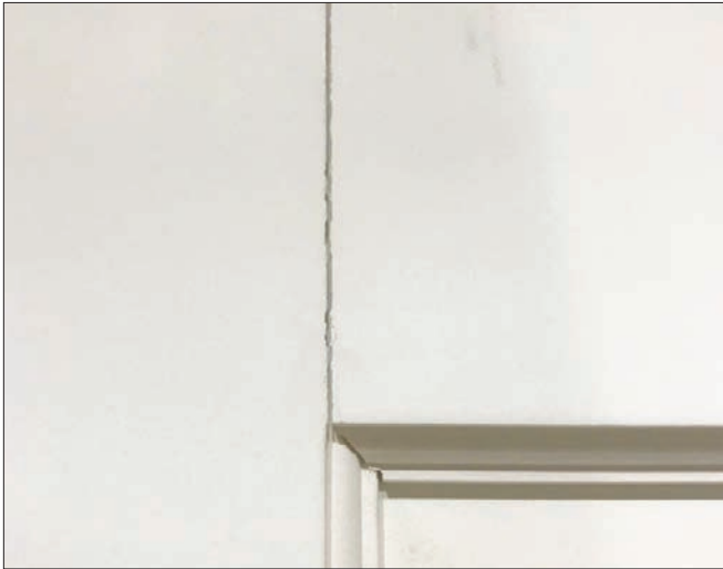
Stile and Rail Separation (Wood Door)
