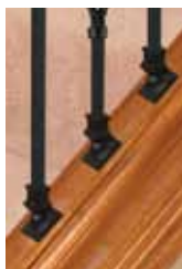
Kneewall Stair Bottom Connection
