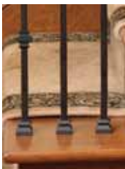
Open Tread Bottom Connection
